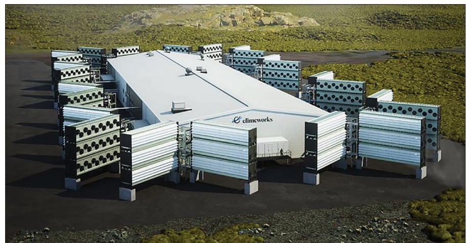
Figure 3. ClimeWorks Mammoth S-DAC project. Modular Solid Direct Air Capture technology being applied at the 36,000 t/yr plant now under construction in Iceland is a 9:1 scale-up of company’s Orca project already in operation, also in Iceland. Source: ClimeWorks.
